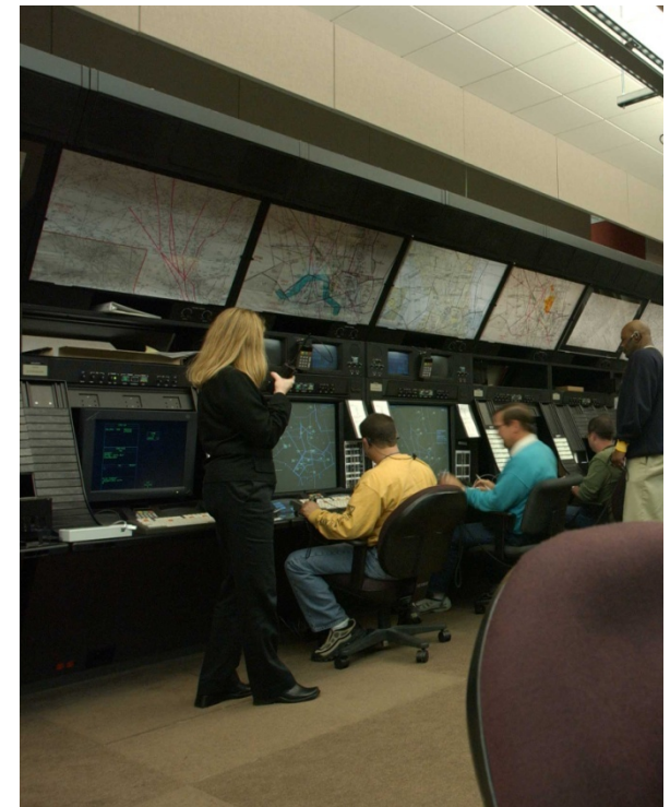
Washington Air Route Traffic Control Center (ARTCC)
