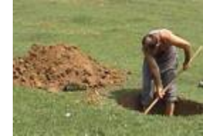
digging a hole
